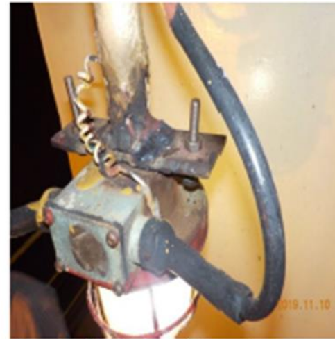
Repaired light foundation at nav. deck
